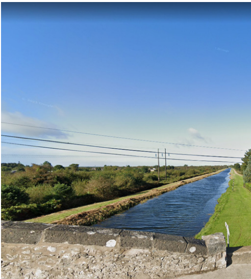
View from Derrymullen (Bond) bridge (west)
