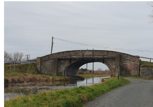
3. Derrymullen (Bond) Bridge
