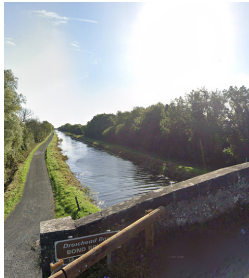
View from Derrymullen (Bond) bridge (east)
